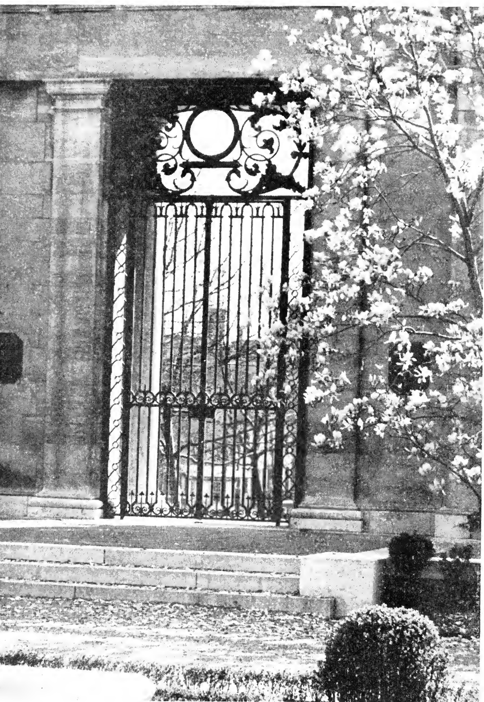
Facade of Rodin Museum Replica of the Musee Rodin, at Meudon, France
